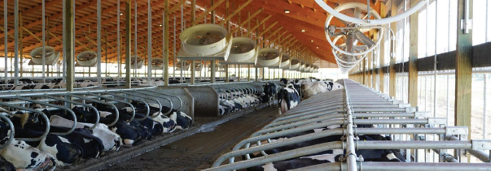
Utilize a high efficiency motor and cash in on environmental rebates with energy savings. This fan can work in a variety of barn ventilation strategies but works particularly well in naturally ventilated barns to boost air circulation.
